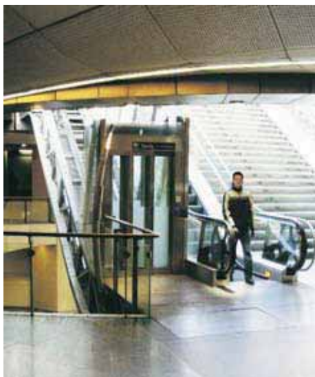
ST. LAZAIRE STATION - PARIS Inclined lift in public service with constant incline Rated load 630 kg n° 2 front landings Incline 30° Travel 8.3 m
