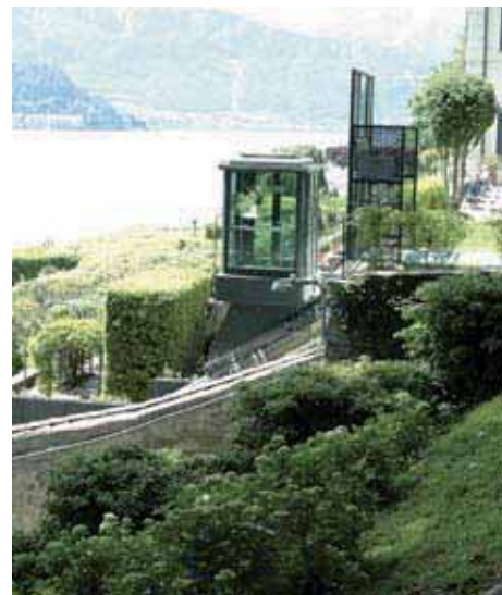
VILLA CARLOTTA BOTANIC GARDENS COMO LAKE Inclined lift with constant incline and front landings Rated load 1000 kg n° 2 opposite front stops Incline 26° Travel 23 m
