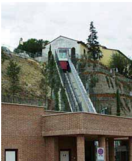
LORETO SANCTUARY - LORETO Inclined lift in public service Rated load 2250 kg n° 2 stops in line Incline 29° Travel 47 m
