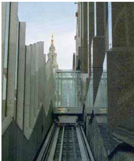
MILLENIUM BRIDGE - LONDON Inclined lift with front landing Rated load 700 kg n° 2 opposite stops Incline 14° Travel 27 m
