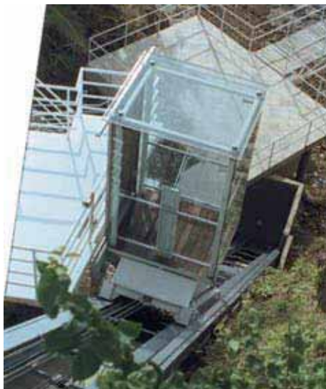
INCLINED LIFT WITH CONSTANT INCLINE Rated load 450 kg n° 3 stops in line Incline 30° Total travel 22 m
