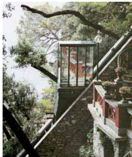
INCLINED LIFT WITH CONSTANT INCLINE Rated load 630 kg n° 3 stops in line Constant incline 56° Travel 40 m
