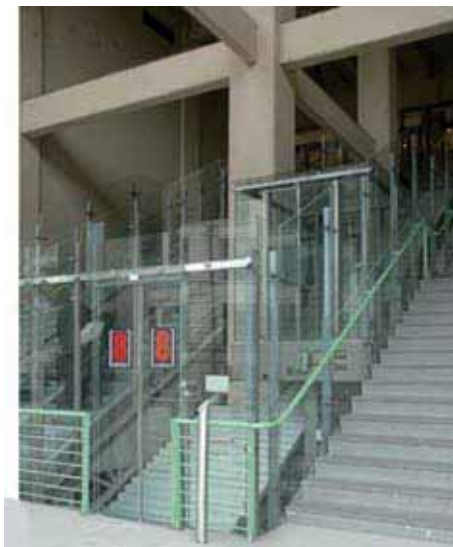
LINGOTTO EXHIBITION CENTER - TURIN Inclined hydraulic lifts with front landings Single automatic operation Rated load 1000 kg n° 2 opposite front stops Incline 30° Travel 15 m
