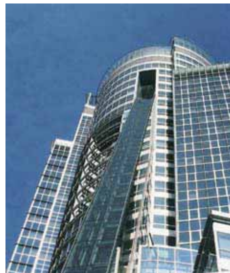
TELECOM TOWER - WARSAW Inclined lift with constant incline Rated load 2500 kg Speed 1.6 m/s n° 28 front stops Incline 78° Travel 105 m Simplex collective operation
