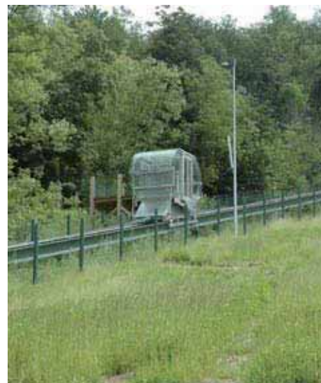
PINO TORINESE ASTRONOMICAL OBSERVATORY - TURIN Inclined lift with constant incline Rated load 2500 kg n° 2 opposite stops Incline 14° travel 197 m
