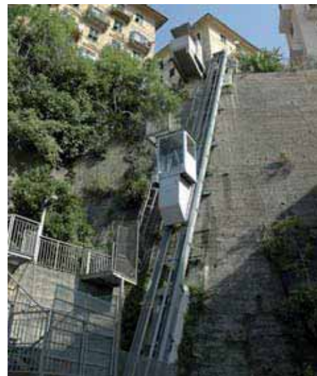
AVEZZANA HILL - GENOVA Inclined lift with constant incline Rated load 630 kg n° 4 stops in line Incline 68° Travel 32 m
